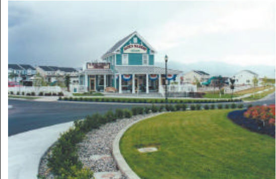
Jack's Market, Stansbury Park, Tooele County with an accessory dwelling unit above the retail space below.
