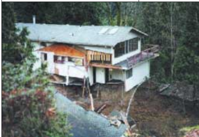
Slope failure claimed 60 homes in Kelso, Washington, in 1998.
