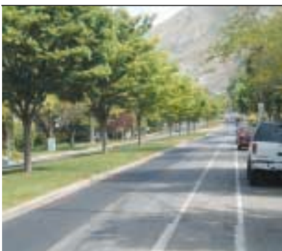
Figure 2: A major residential street located in Salt Lake City providing center medians, street trees, on-street parking and bike lanes.
